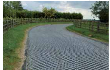
TECHPAVE HD80 interlocks with adjacent pavers
